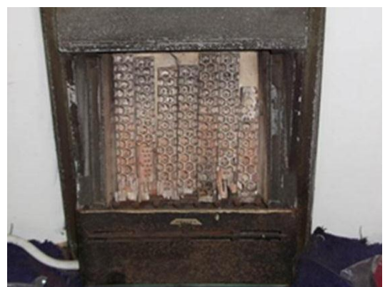
An old, unsafe gas fire that we disconnected from live gas supply.
